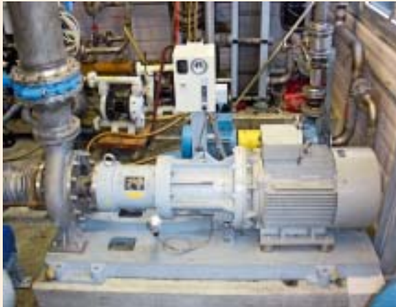
Uncomplicated: retrofitting to the horizontal magnet-coupled MPCH DryRun centrifugal pump manufactured by Bungartz
